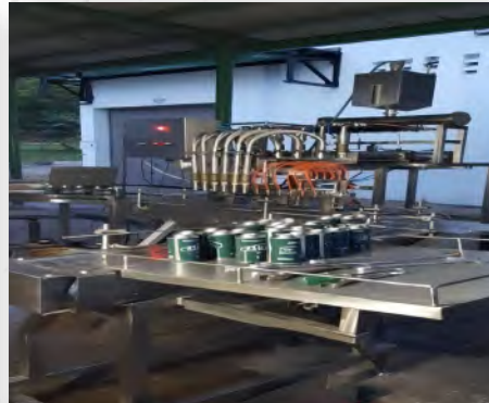
AUTOMATED HARDENER FILLING STATION 2
